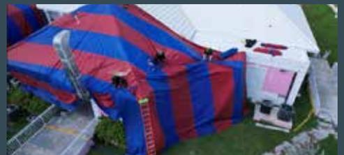
The tent you often see is what creates the seal to keep the gas inside, or in some circumstances where a particular roof with specialised construction is in place, we can " Tape & Seal " plastic sheets from the inside of the property and create a seal for no gas to escape. (also available for fragile roof tiles).
