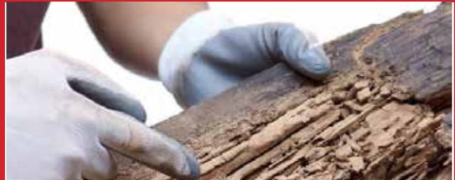
A fumigation is the only way to exterminate all. Fumigation works by creating an environment where a specialist gas is injected into the property and it can't escape ( or escape quickly ) allowing a build up in concentration of gas, where it gets to a point where it kills everything inside the property.
